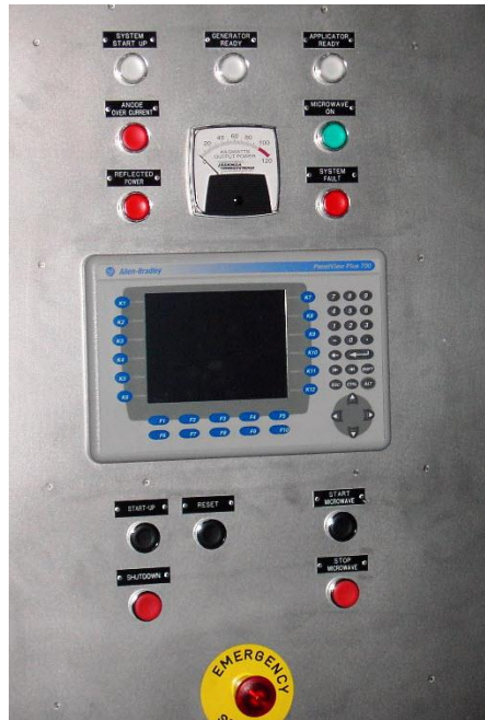
The Generator Control Panel with the PanelView Operator interface is shown above.
