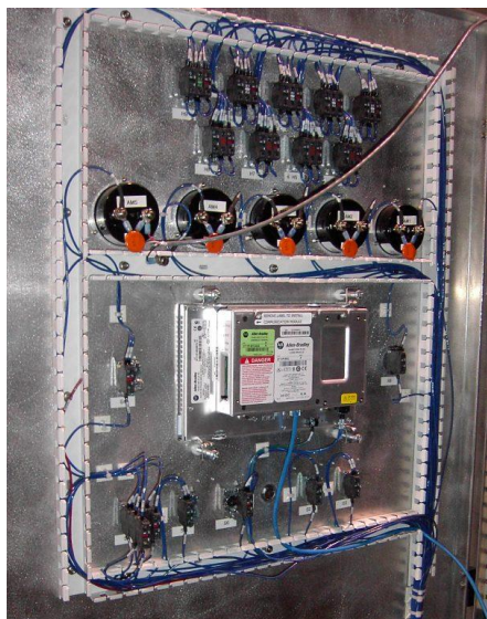
The above pictures show the rear of the Main Control Panel on the left and the PLC and Control Relay Panel on the right.
